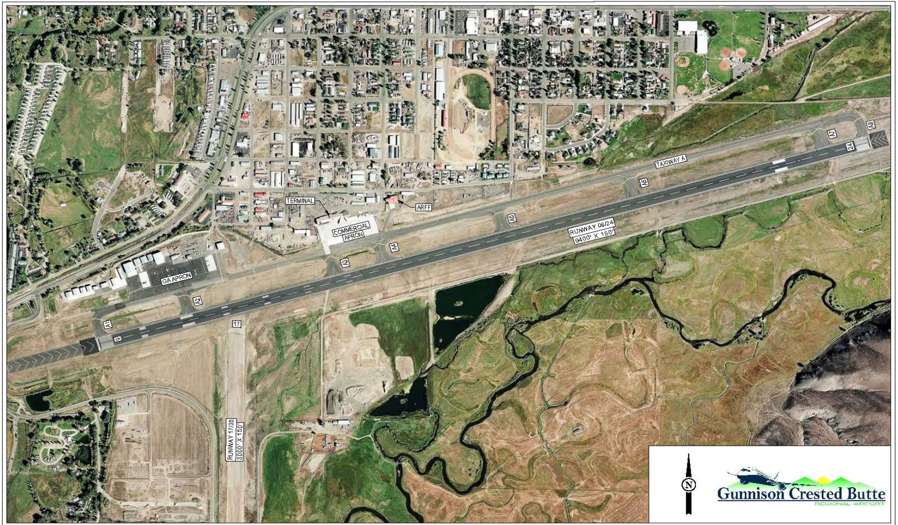
FIGURE 1-1 GUNNISON CRESTED BUTTE REGIONAL AIRPORT
