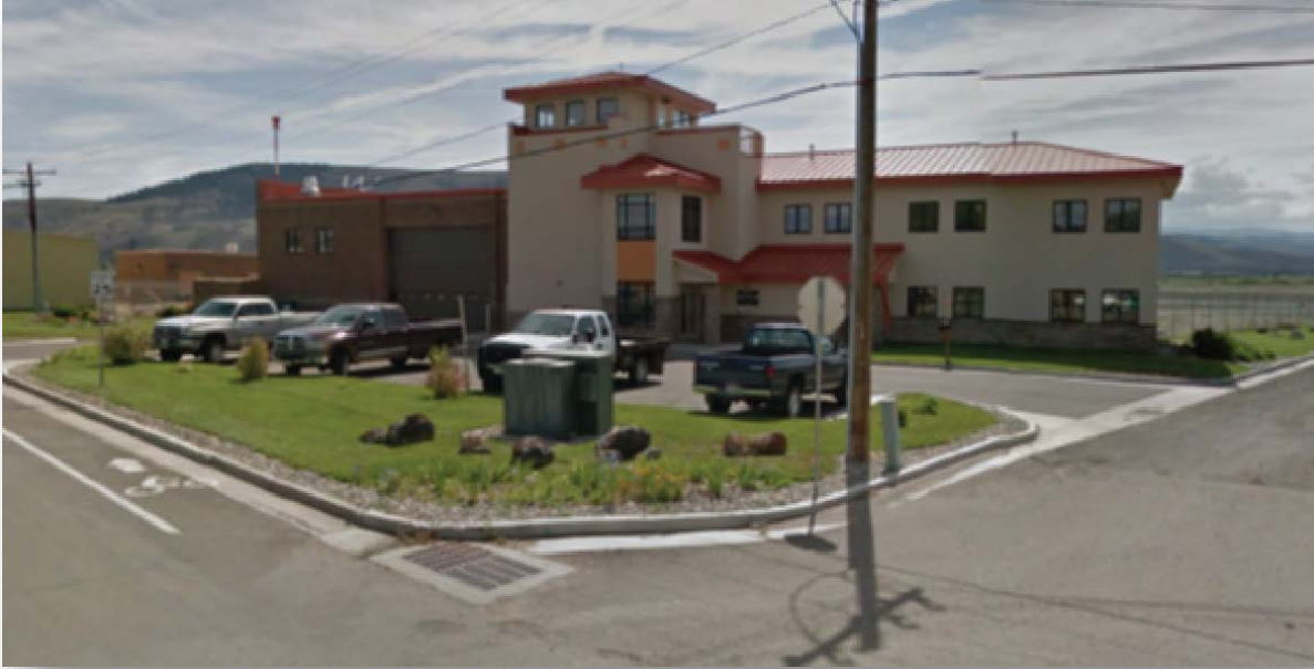
FIGURE 1-37 ARFF AND SRE STORAGE BUILDING AND AIRPORT ADMIN OFFICES
