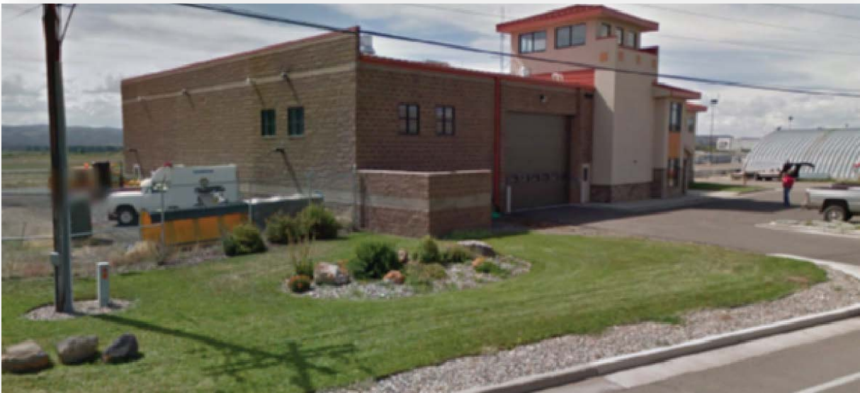
FIGURE 1-38 ARFF AND SRE STORAGE BUILDING AND AIRPORT ADMIN OFFICES
